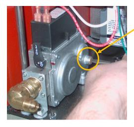
Remove the adjustment screw cap from the gas valve using a short "stubby" flat head screwdriver.
