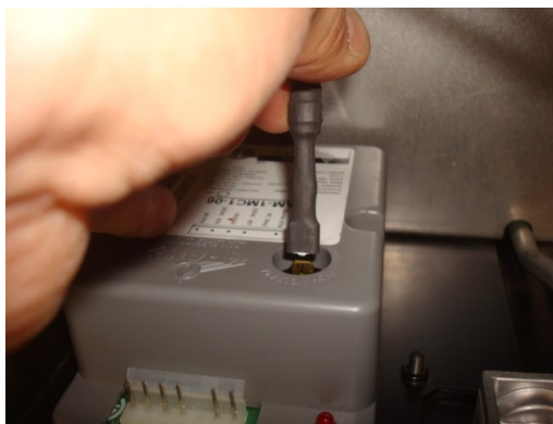
Disconnect high voltage cable
