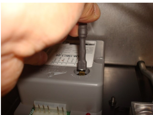
Connect high voltage cable
